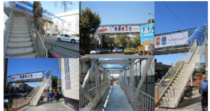
Fig.6. Pedestrian Bridge in CBD
